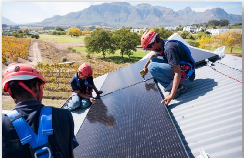
Figure 2: Installation of solar panels
